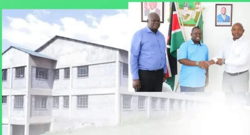
Construction of Stalled Shamakhubu Hospital Resumes early 2024 after MPs intervention through the office of the governor
